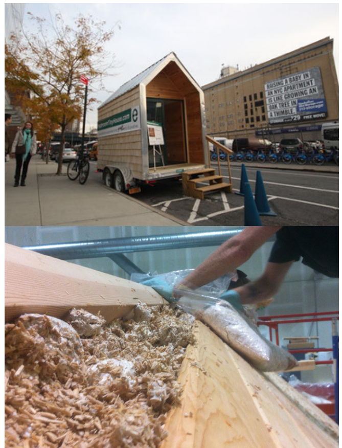
FIGURE 218 FILLING THE WALL CAVITY OF THE TINY HOUSE WITH MYCELIUM COMPOSITE, 2013 (WWW.MUSHROOMTINYHOUSE.COM)
