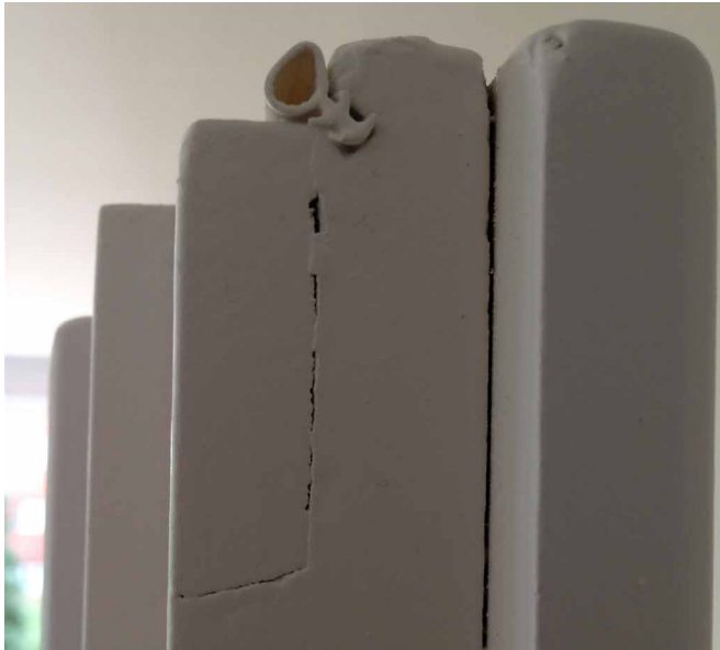
FIG. 5.28 Sash frame with new sealing: a) Image and b) schematic drawing / Photo: S. Rexroth
