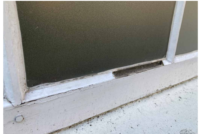
FIG. 5.18 Putty in wooden windowframe (in need of repair) / Photo: W. J. Quist
