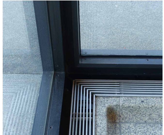
FIG. 5.40 New National Gallery, Berlin: New facade with a single glazing in a thermally non-separated construction / Photo: F. May
