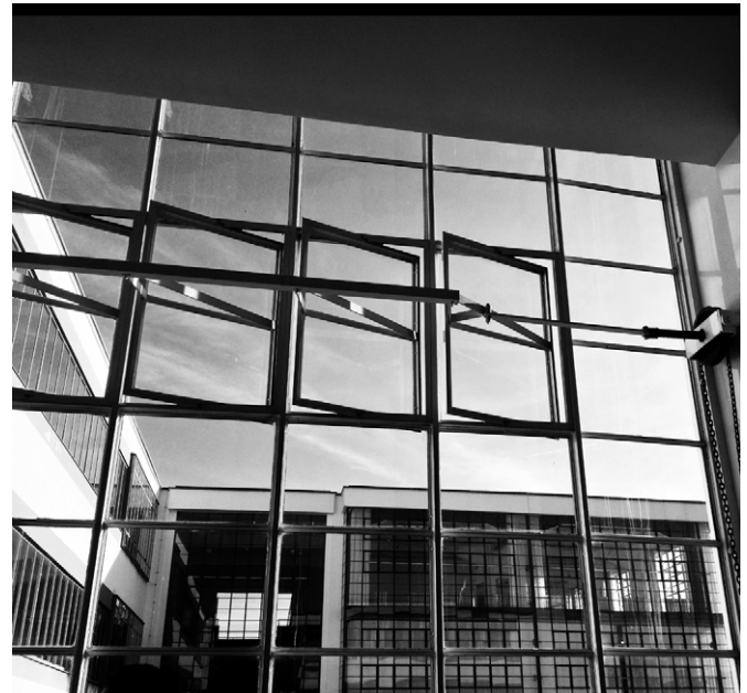
FIG. 5.8 Bauhaus Dessau, staircase, office and workshop glazings were originally using polished plate glass to achieve a precise and industrial look / Photo: pixy.org
