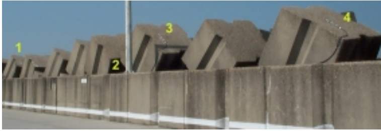
Figure 4.21: Wave detectors on the crest of the Zeebrugge breakwater.
