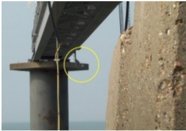
Figure 4.19: Video camera suspended on the measuring jetty and directed towards the armour layer units of the breakwater.
