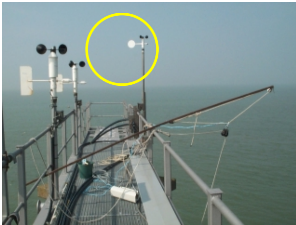
Figure 4.18: Anemometers placed on the measuring jetty provide wind data (wind speed v_s and wind blowing direction \beta ).
