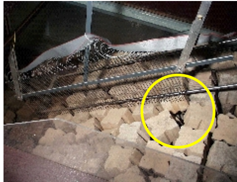
Figure 5.12: Indication of a hole underneath the upper 10 electrodes of the run-up gauge.
