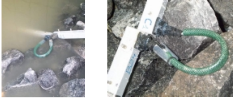
Figure 5.64: Connection cable between run-up gauges protected by a piece of garden hose.
