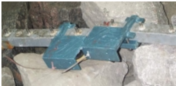
Figure 5.65: Shield protecting the connection of the cables to the gauges.
