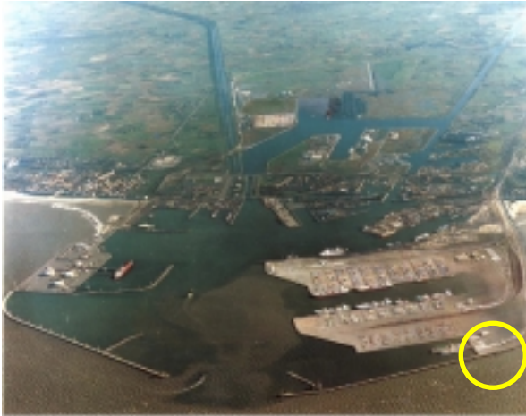
Figure 4.2: Aerial view on Zeebrugge outer harbour with indication of the measuring site (photo: MBZ).
