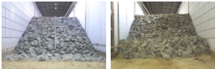
Figure 5.56: View on (a) seaward slope and (b) landward slope of the breakwater.
