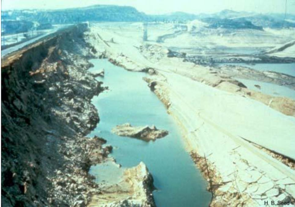
**Figure 2.3: Liquefaction flow failure at the Lower San Fernando Dam due to the 1971 San Fernando earthquake, after lowering the reservoir**
