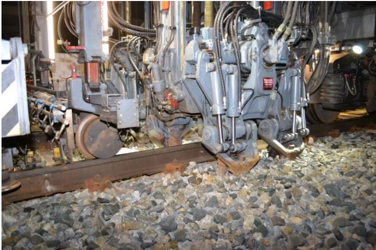
Figure 11. Tamping in a transition zone.
