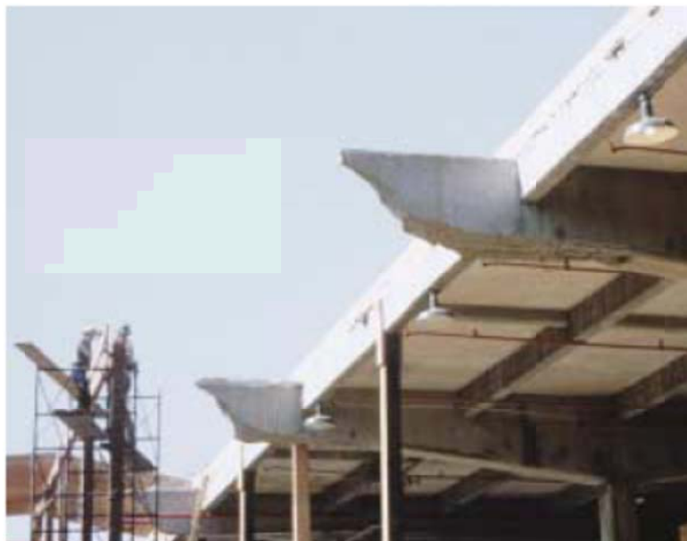
Fig. 3.62: Shear failure of 900mm deep beams in the Air Force Warehouse, Shelby, OH (Lubell, et al. 2004).
