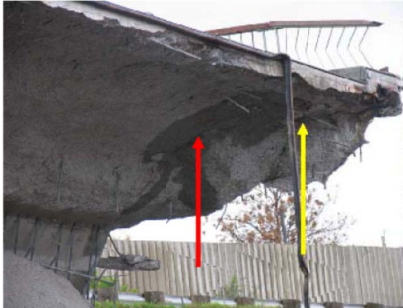
Fig. 2.5: Shear failure of the Laval bridge (Massicotte, 2007).
