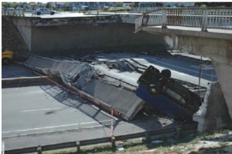
Fig. 2.4: Collapse of the de la Concorde overpass (Wood, 2008).
