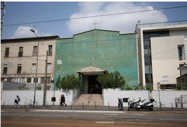
Figure 1 – The southern façade of St. Pio X Church (Case Study 1), facing Piazza Leonardo da Vinci square.
