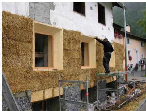
Fig. 9 Insulating with straw - bio-based alternatives for futureproofing buildings 33
