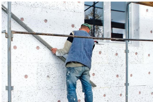
Fig. 8 Adding Styrofoam insulation - Standard practice in Poland. (Murator.pl) 32
