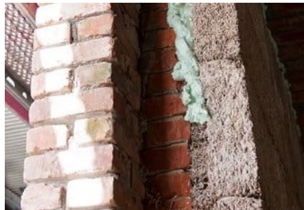
Fig. 2 Farmhouse renovation – additional interior insulation using hempcrete. (HempBuild, 2024)
