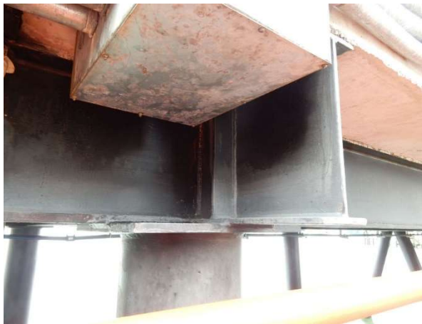
Figure C-7: Rigid column-beam connection
