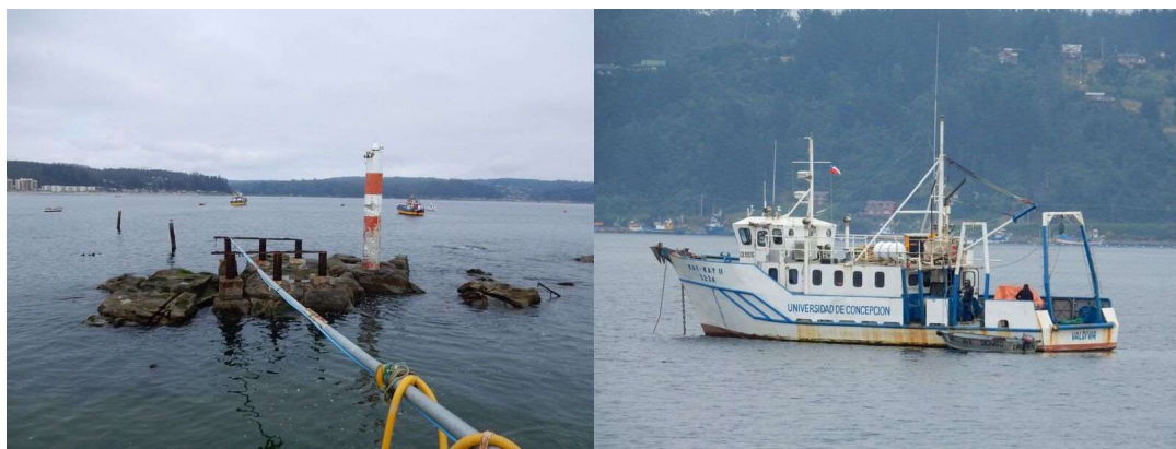
Figure Map 3 D: Existing piles from previous jetty
