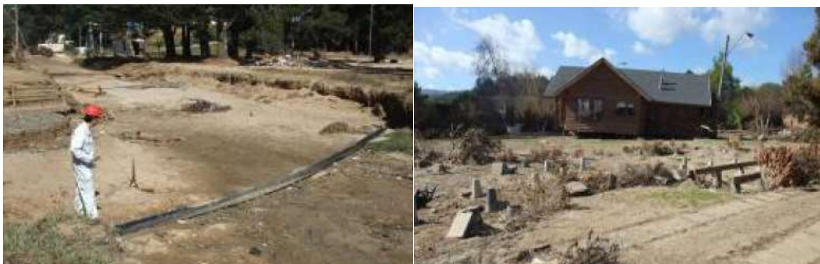
Figure A-12: (Left) Exposure of buried lifeline due to tsunami erosion. (Right) House lifted from foundation and moved inland.
