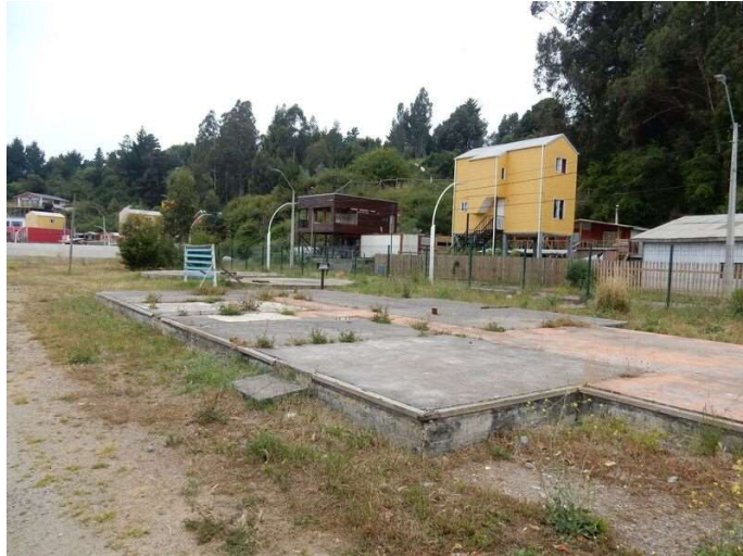
Figure Map 2 A: Concrete remains of shallow foundation for stay-over cabins. Potential redevelopment site
