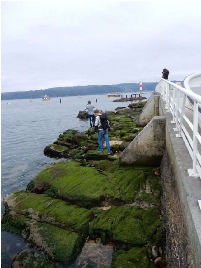
Figure Map 3 A: Abutment sea-side with concrete protrusions and foundation rock outcrops
