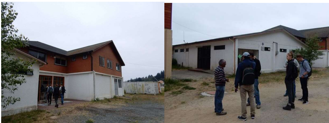
Figure Map 2 G: (Left) Building with research facilities for organisations, including INCAR
