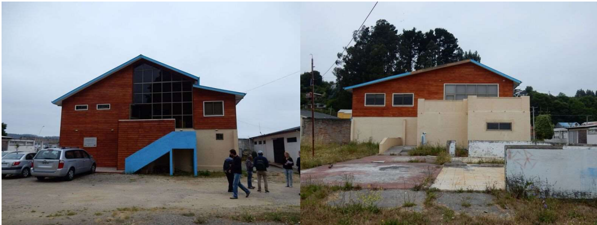
Figure Map 2 B: Building completed in 2014 (Left: Entrance side, Right: Sea-side)
