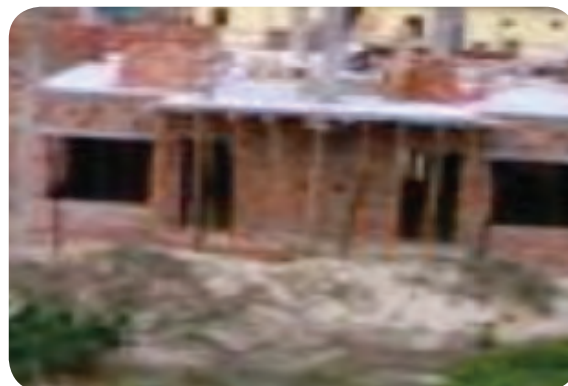
Figure 15. Construction on the dune, Digha, West Bengal
