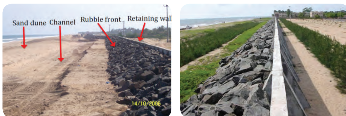
Figure 13. Sand dune and seawall at Kalpakkam, Tamil Nadu
