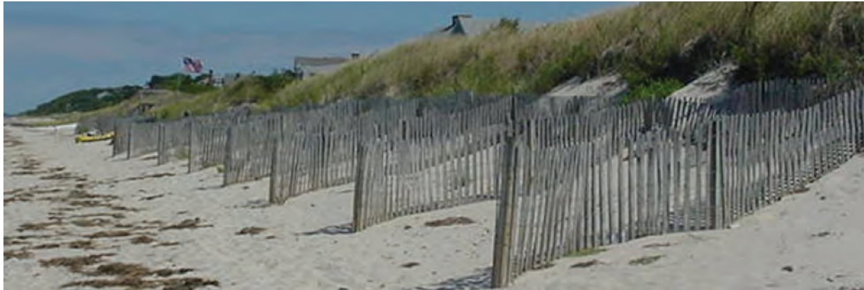
Figure 6. Sand fencing used to help trap sand and stabilize dunes
