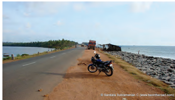
Figure 2. Coastal road in Maravanthe
