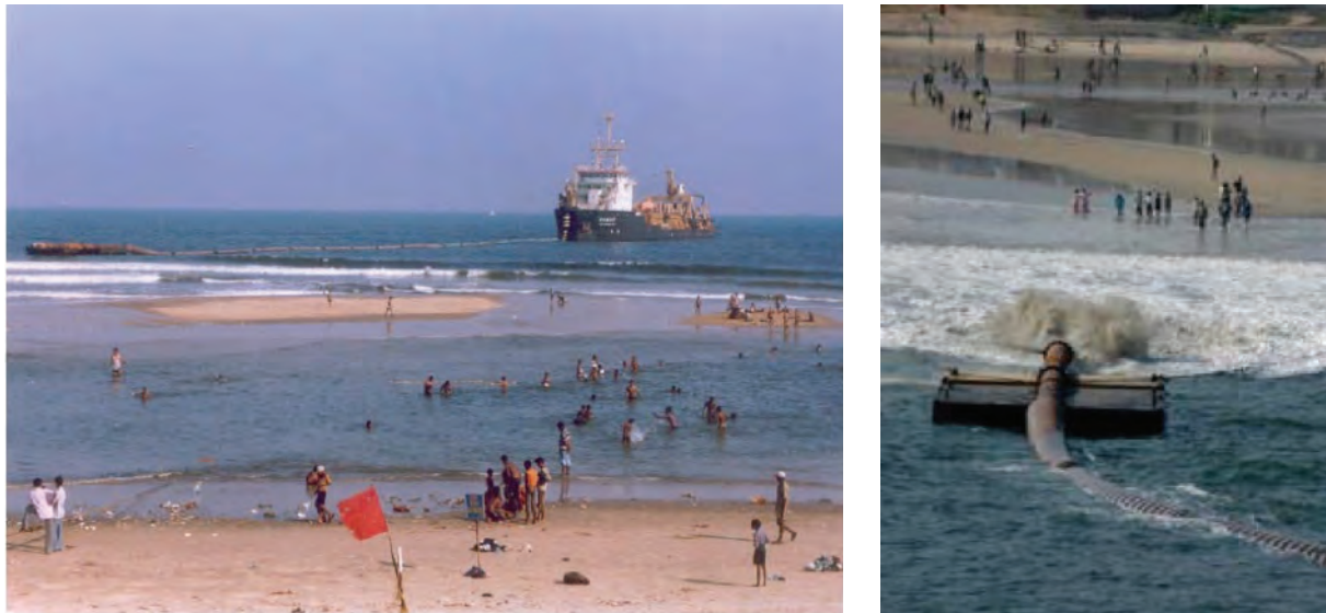
Figure 23. Beach nourishment through a rainbow pontoon at Visakhapatnam Port
