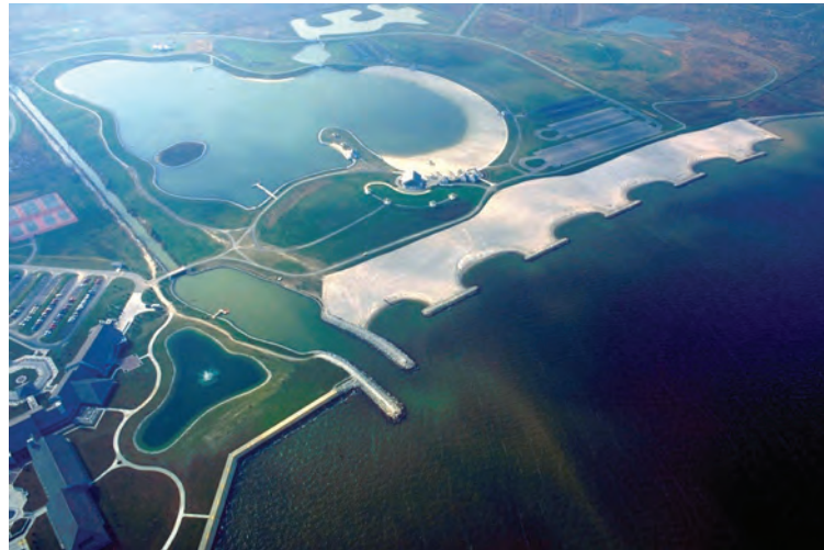
Figure 16. Maumee Bay State Park (United States) showing a nourishment program combined with offshore breakwaters
