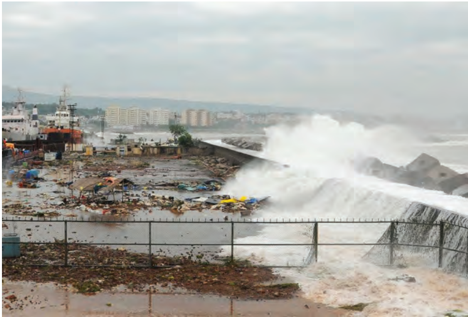
Figure 8. Existing rock seawalls in the Visakhapatnam district are already some 15m high, but are still overtopped during cyclones
