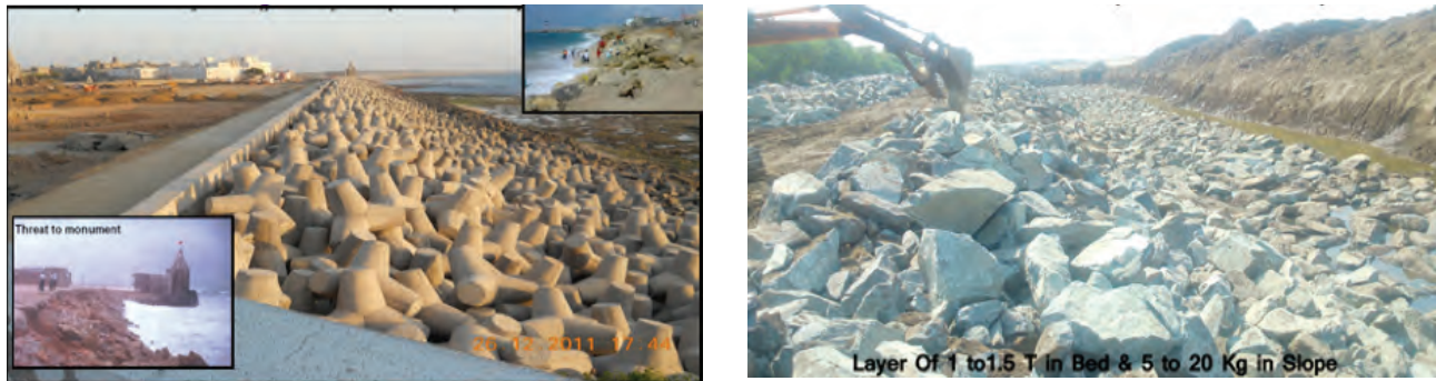
Figure 7. Seawalls in Gujarat, (left) Dwaraka and (right) Dumas, with low gradient and long toe
