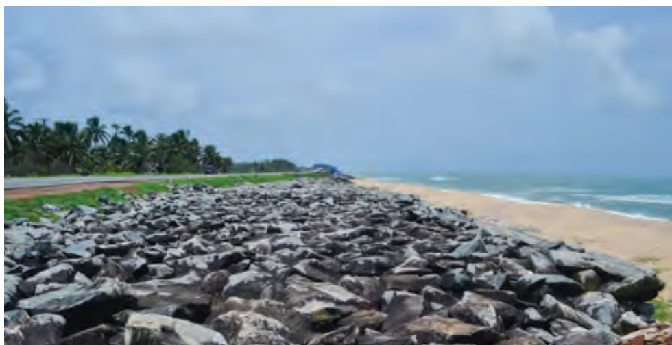
Figure 3. Rock dumping to protect coastline
