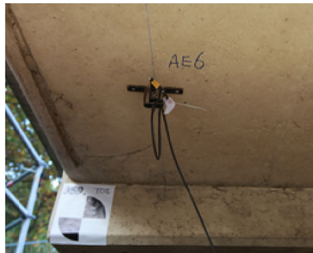
Figure 21. Installation of AE sensor in a proof load test in the Netherlands.
