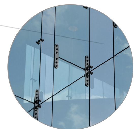
Structural glass fins stability | view
