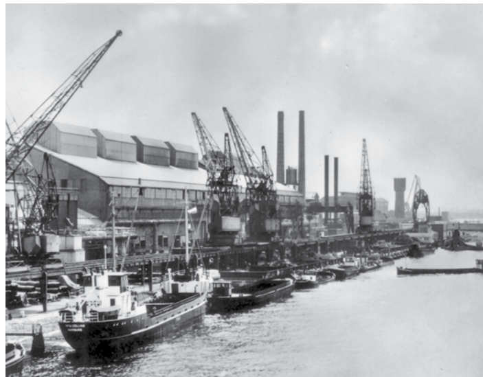
Figure 17: View of the loading docks of Nedstaal. The smelter building is in the back. (HSA, 2024).
