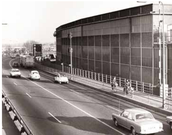
Figure 16: View of the wire mill building from the "Bridge over the North" - the first facade seen from that road when entering Alblasterdam (Bridge Management Information Department, 1970).
