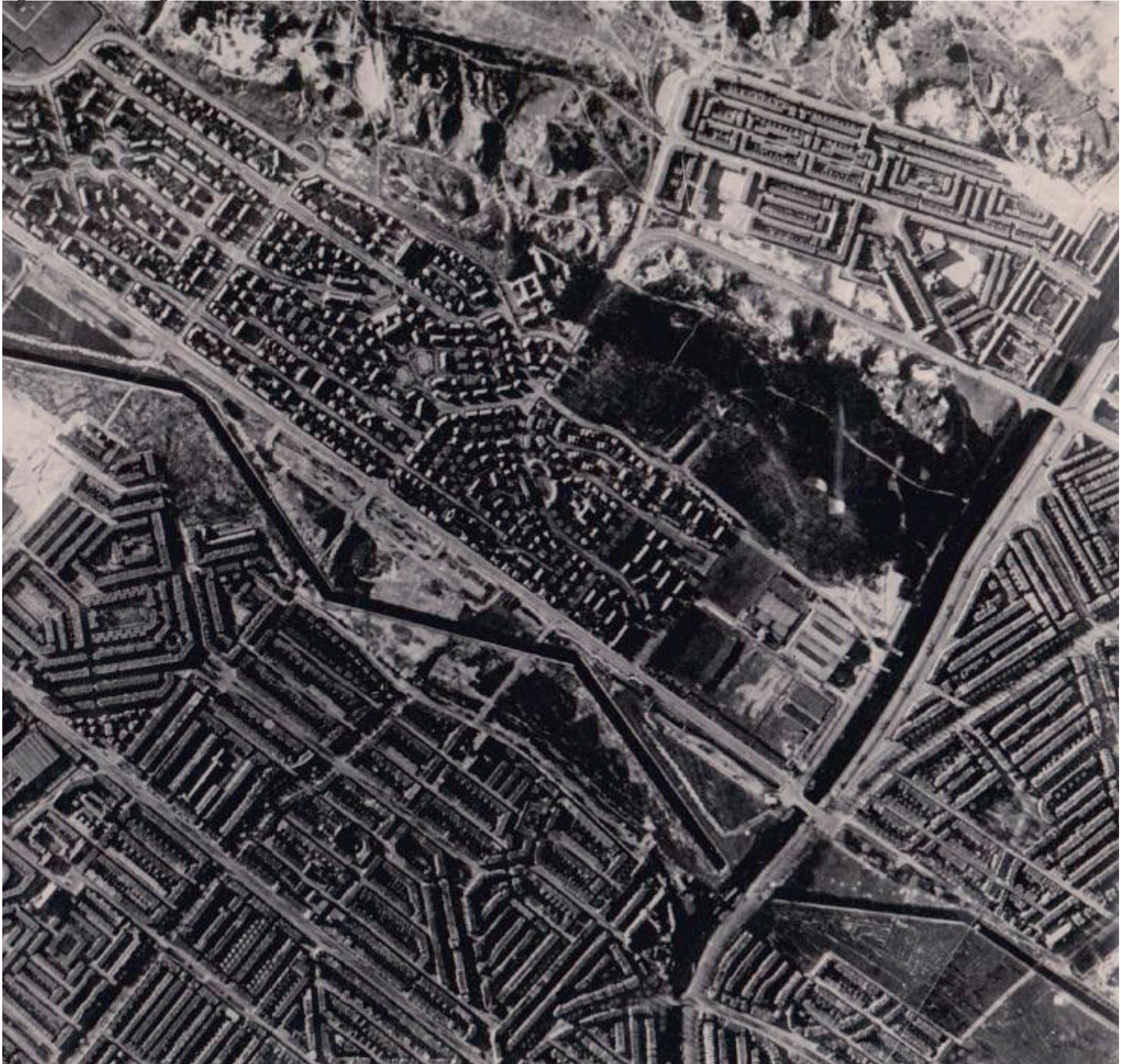
Figure 1.4 Damage Atlantikwall Verversingskanaal
