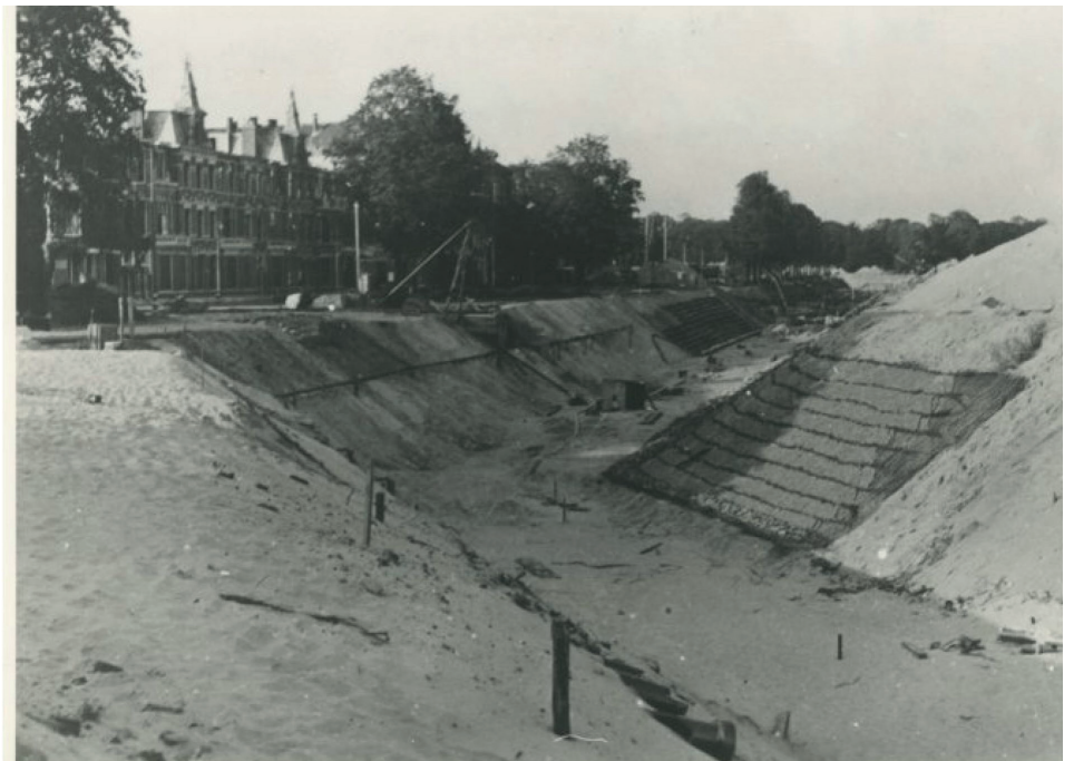
Figure 5.13 Construction of anti-tank ditch Stadhoudersplein
