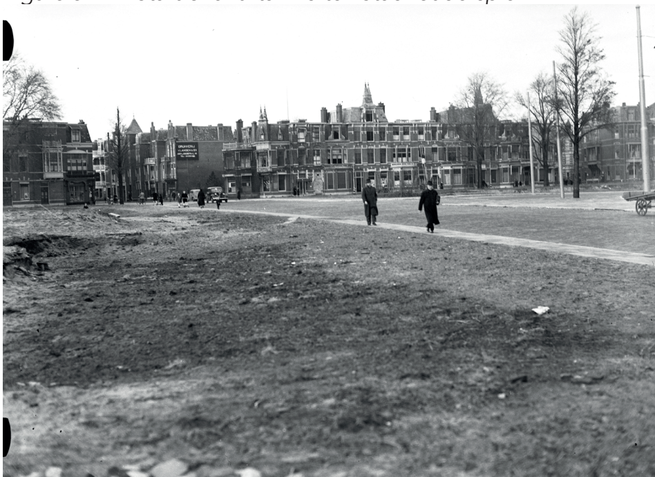
Figure 5.12 Start of anti-tank ditch Stadhoudersplein
