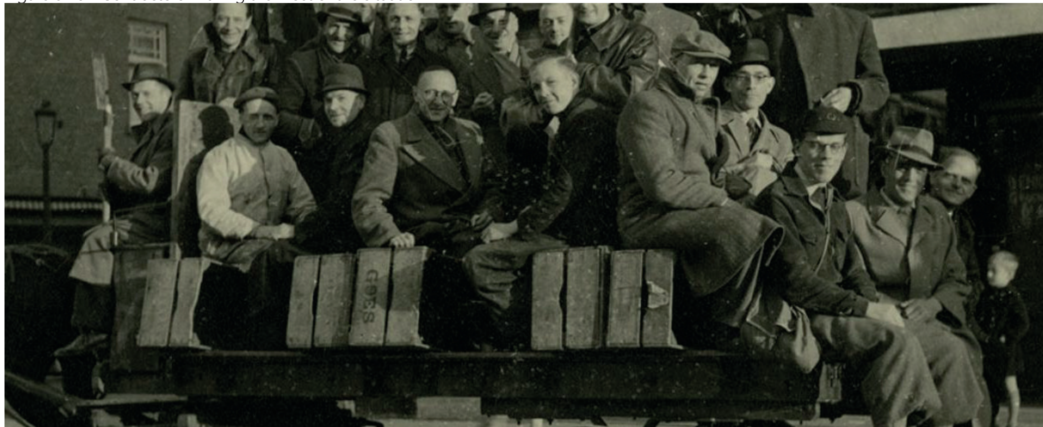
Figure 5.25 Contractors 'making the most of the situation'
