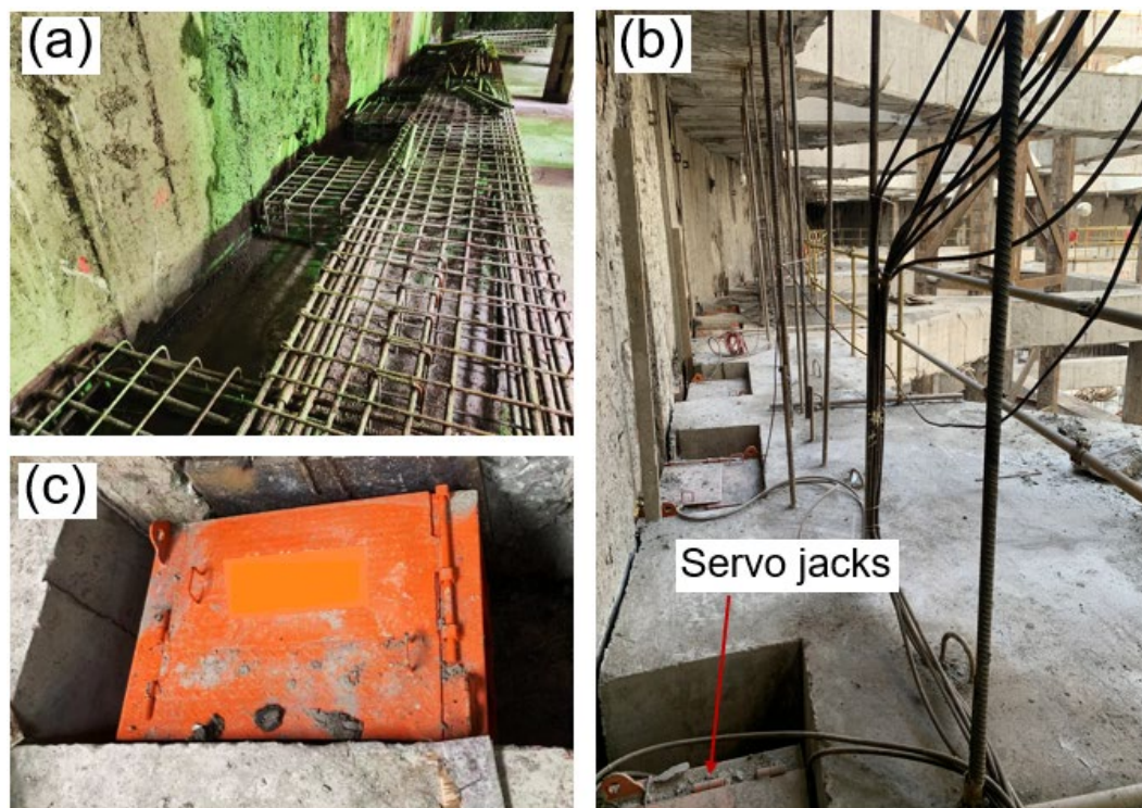
Figure 6. Bracing structure design of the Z3 with servo concrete struts: (a) reinforcement cage of purlin; (b) field construction of servo RC struts; and (c) servo-hydraulic jack.
