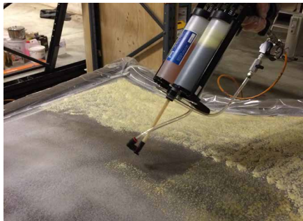
FIGURE 6.16 Applying the HDPU
