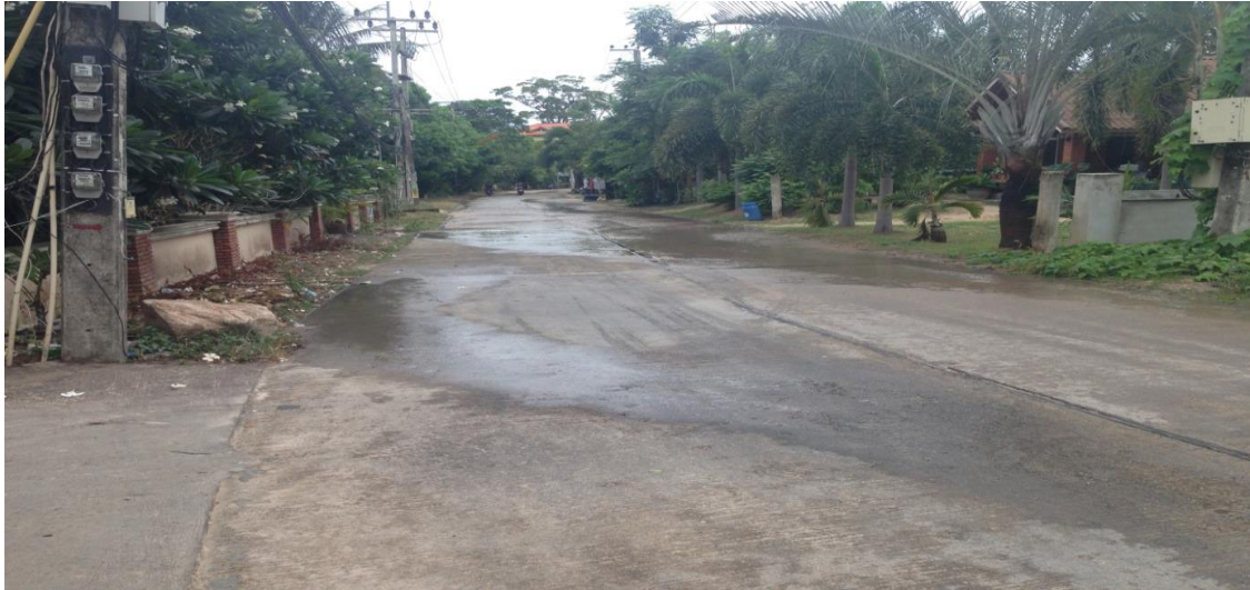
Figure 15: Runoff from a road without trenches
