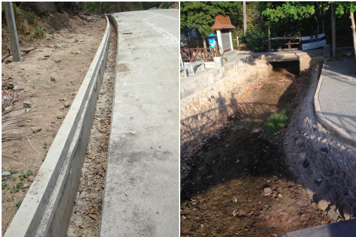
Figure 16: New road with trench (Left) - Figure 17: Drainage canal (Right)
