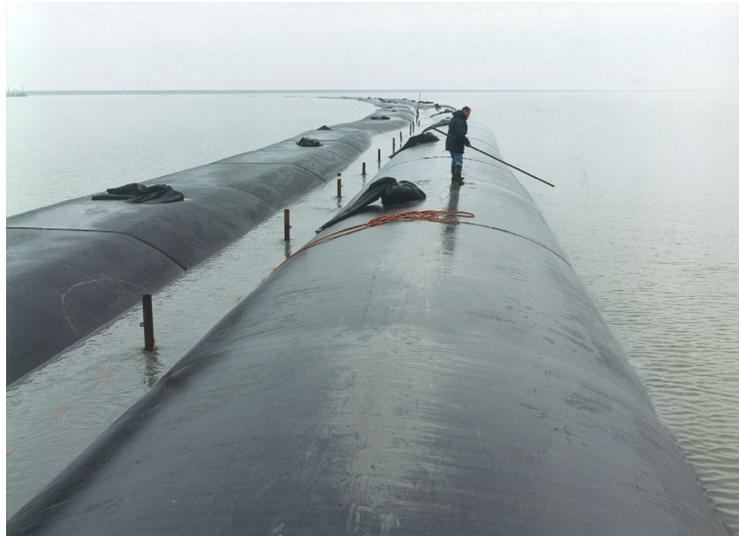
Figure 16. Example of construction of breakwater using geotubes
