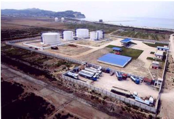
FIGURE 1.5 – OIL PLANT ROMANO-PORT
