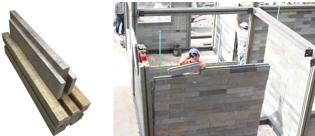
Figure 12 (left) and 13(right). Prefabricated Plastic Building Components by 'Conceptos Plasticos'
