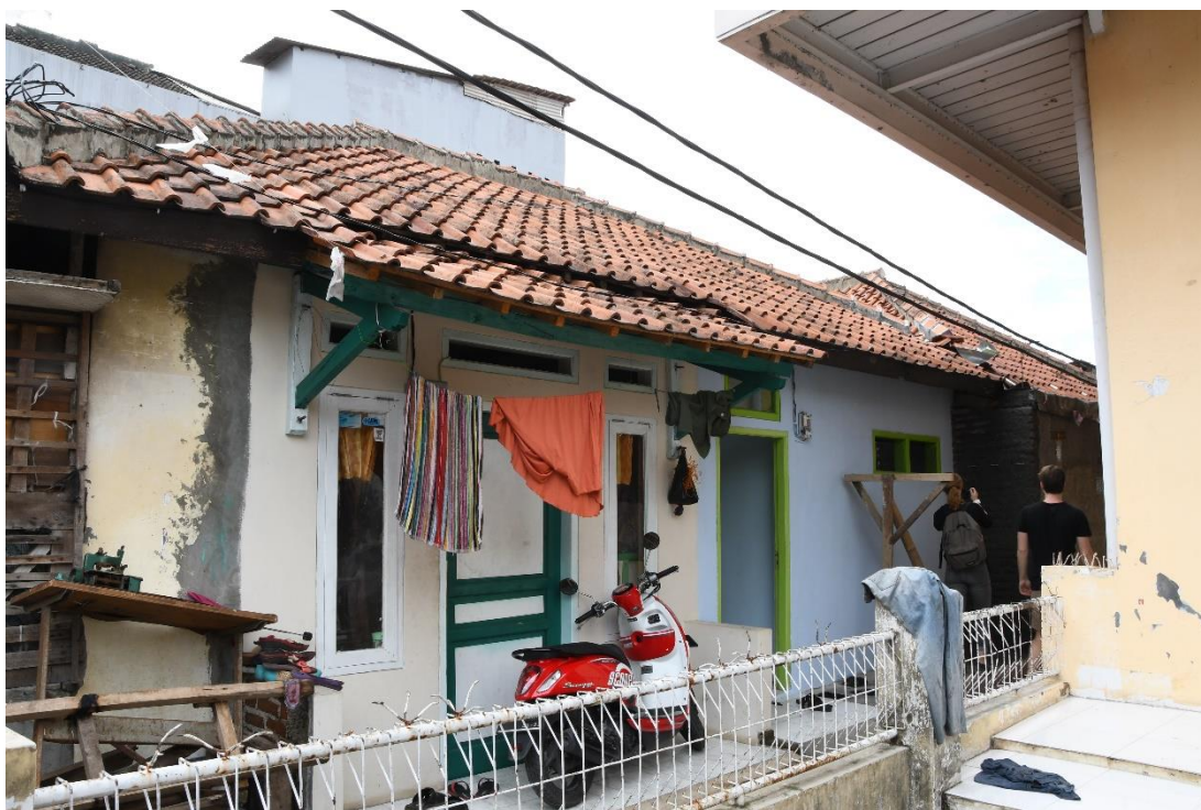
Figure 2. A Typical Kampung House in Cigondawah
