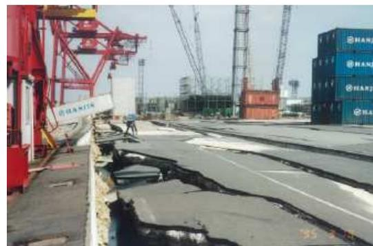
Figure 5-5 Damage Kobe Port due to liquefaction during the 1995 earthquake.
