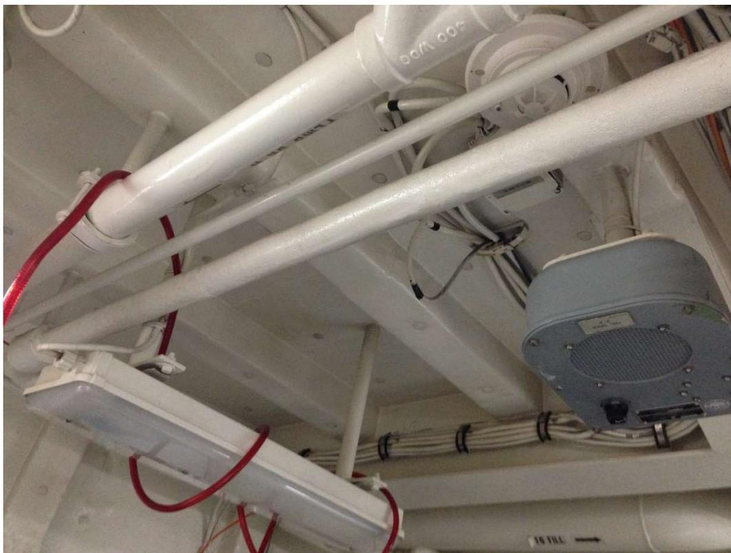
**Figure 6.14 –Inside view of a US Coast Guard Cutter showing insulated primary hull girder structure – relevant to PoD of NDT and difficulties for visual or NDT inspection**
