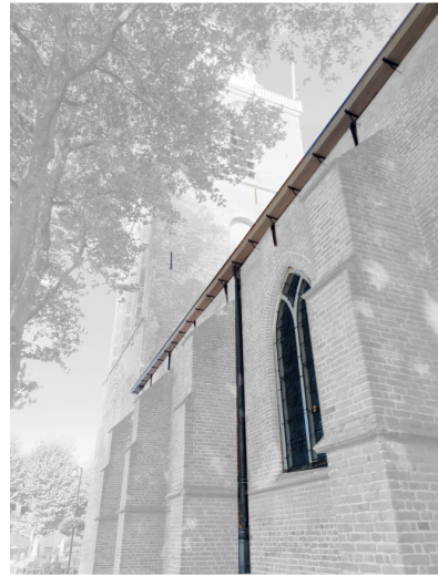
4 floor anchors, rain pipe and windows
