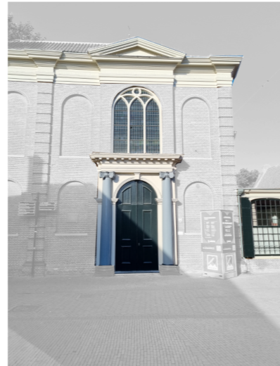
6 Wooden ornaments and window frames
