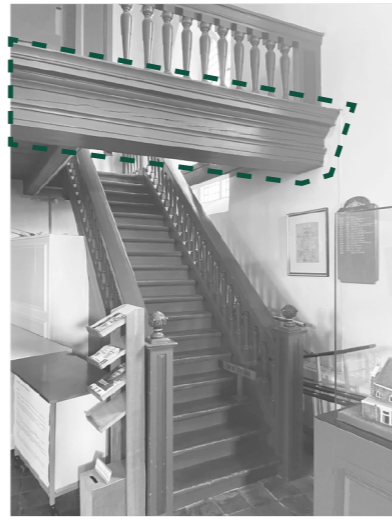
3 Wooden beam supports in wall
