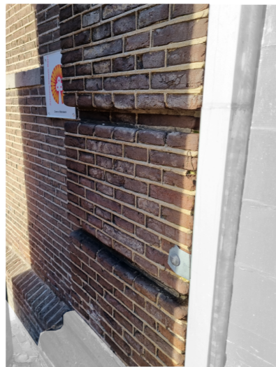
5 Masonry bond east facade
