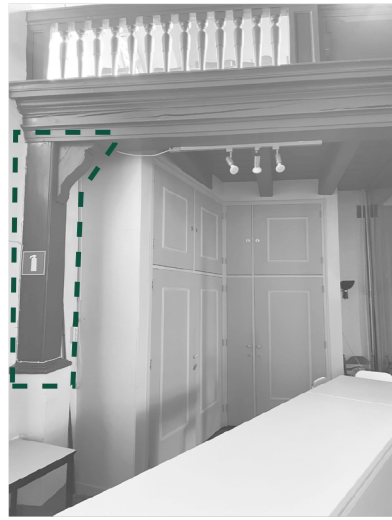
1 Wooden supporting column
