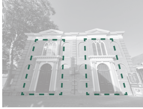
3 East facade facade openings
