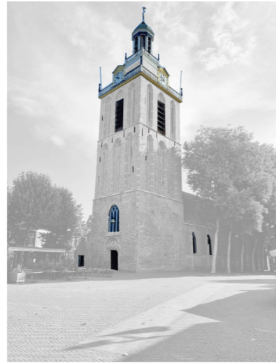
5 Wooden tower elements and iron floor anchors and window frames
