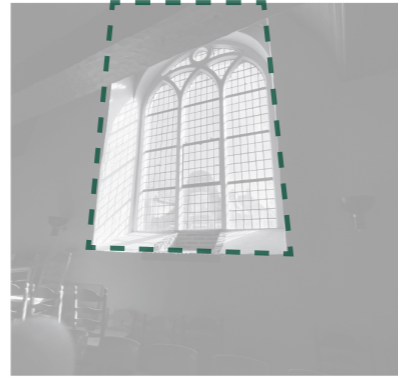
3 East facade window
