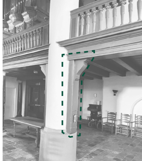
2 Wooden support on pillars
