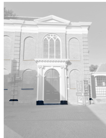
6 Concrete thresholds and pillar feet
