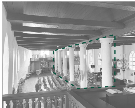
5 Plastered masonry pillars supporting the roof
