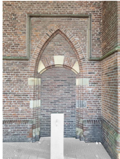
6 Masonry bond and ornaments
