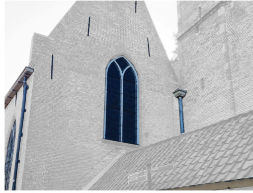
1 floor anchors, rain pipe and windows
