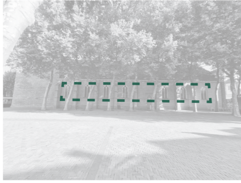
2 South facade facade openings
