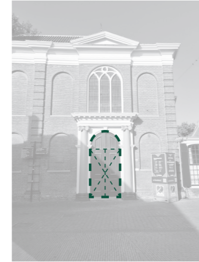
2 Eastern facade entrance
