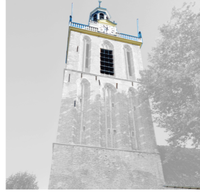
3 Wooden tower elements and iron floor anchors
