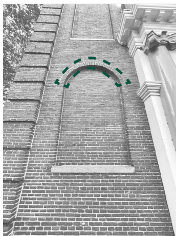
4 Semicircular masonry arch
