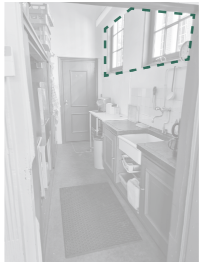
4 Preacher's house kitchen window
