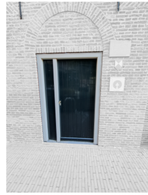
2 Wooden door and window frame
