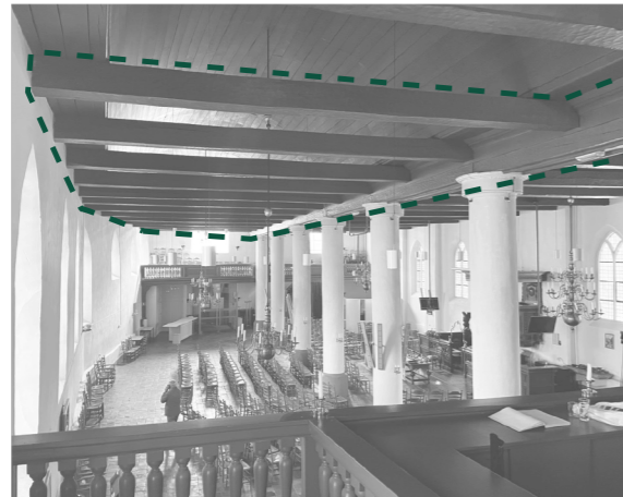
5 Wooden beams supported by pillars
