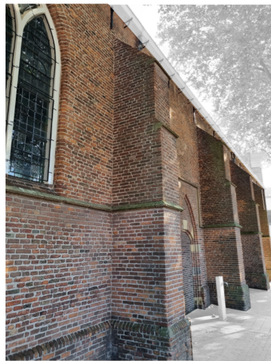
4 Masonry bond buttresses
