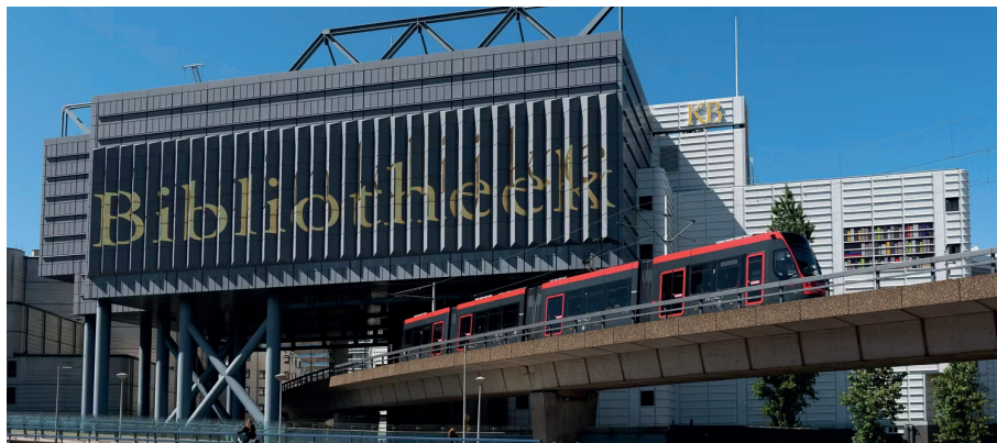
Figure 6 | Building of the KB
