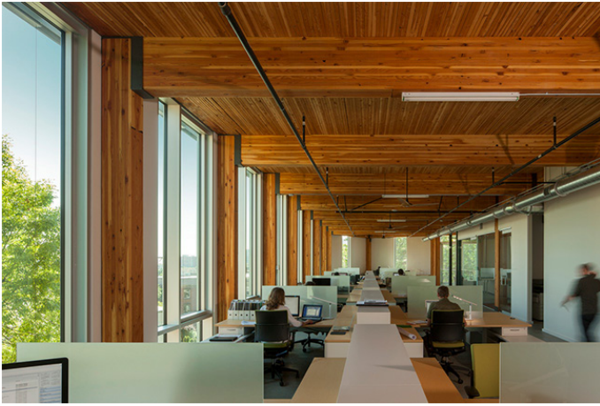
Figure 7 The Bullitt Center timber beams
