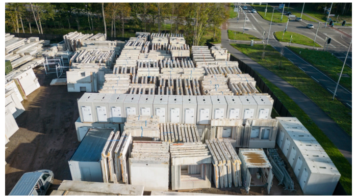
Figure 11 Moved elements Temporary Courthouse Amsterdam
