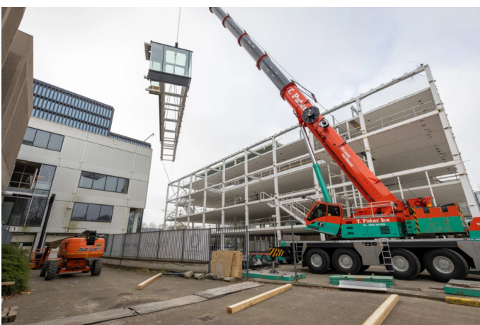
Figure 10 Dismantling of Temporary Courthouse Amsterdam
