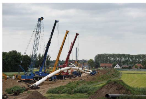
Figure 9 Installation of the 600 m 48-inch gas pipeline (bottom), using a 60-inch flycutter and 48-inch barrel reamer (top) and a 450 tons drilling rig (middle).
