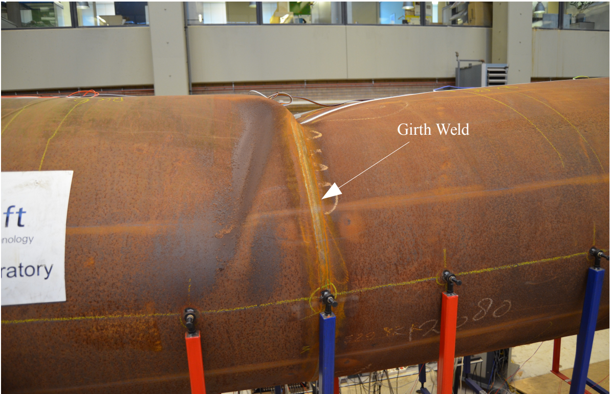
Figure 5: Example of girth weld
