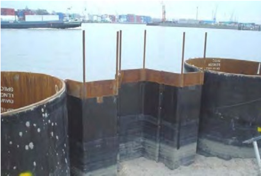
Figure 1: Combined sheet and pile wall
