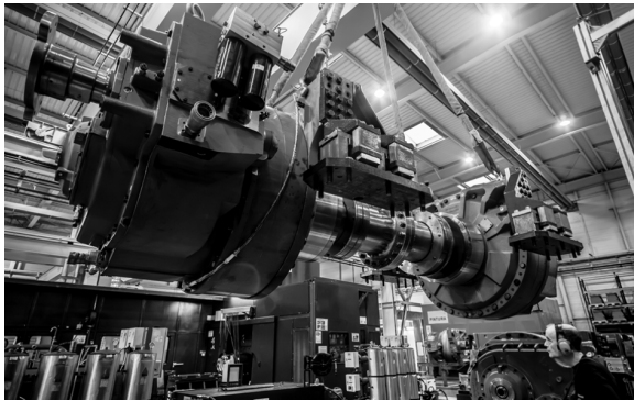
Figure 2. Lift operation of two gearboxes.
