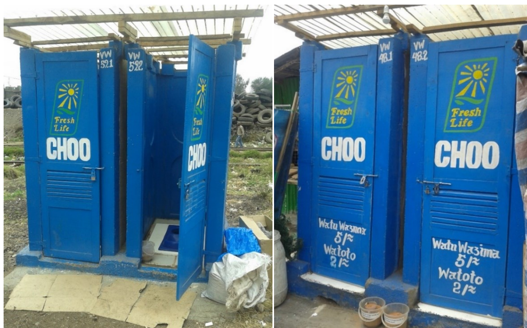
Figure 6-1. Fresh Life ® toilets installed in a slum in Nairobi, Kenya
