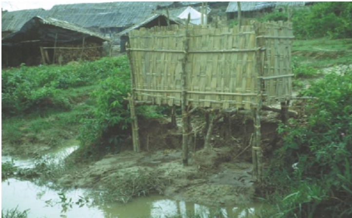
Figure 2-5. Overhung latrine, Bangladesh (Harvey et. al 2002)
