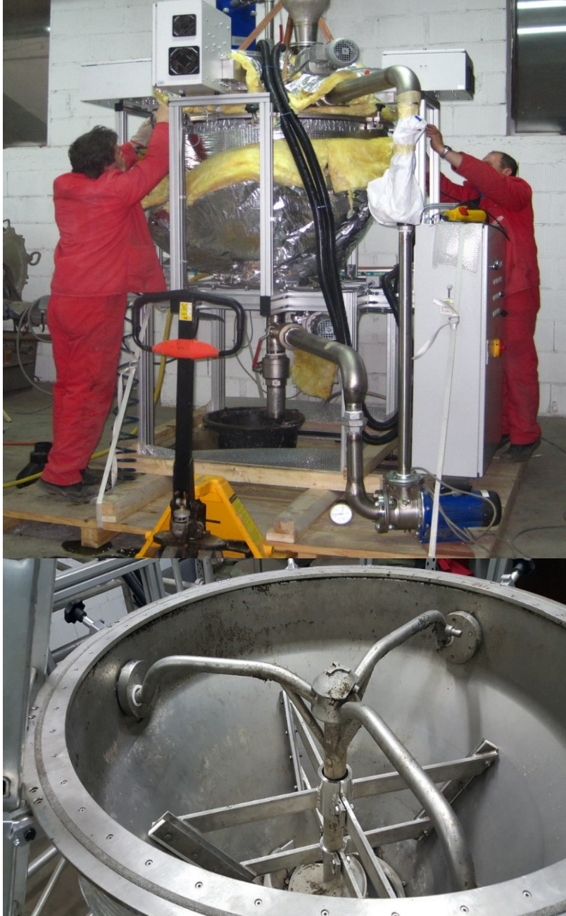
Figure 7-7. Reactor Version 2 with an installed recirculation pump (top) and a mechanical mixer (bottom)
