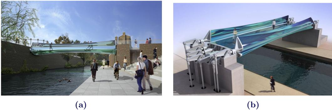
**Figure 2.10:** Glass footbridge consisting of compressed glass sheets, taken from Rinaldi (2014); (a) Impression of the bridge in its surroundings; (b) Introduction of compression force by lever-arm systems;
