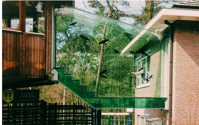
**Figure 2.3:** Second glass bridge in Arnhem, incorporating a glass stairs, taken from Nijse (2003);
