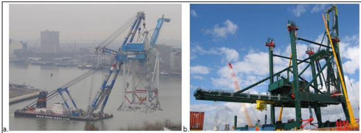
Figure 4.11 a) Placement of crane on rail using a floating crane barge b) Erection of crane on site using strand jacking
