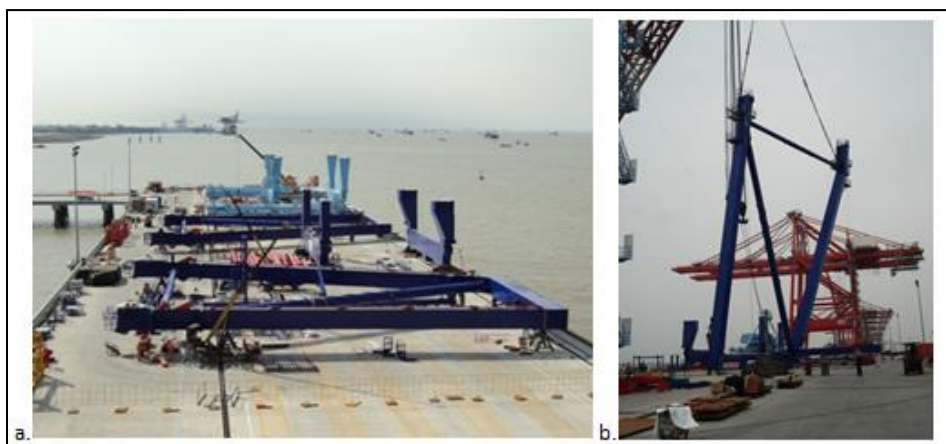
Figure 4.22 a) Horizontal assembly of the side portal b) Lift of the side portal for placement
