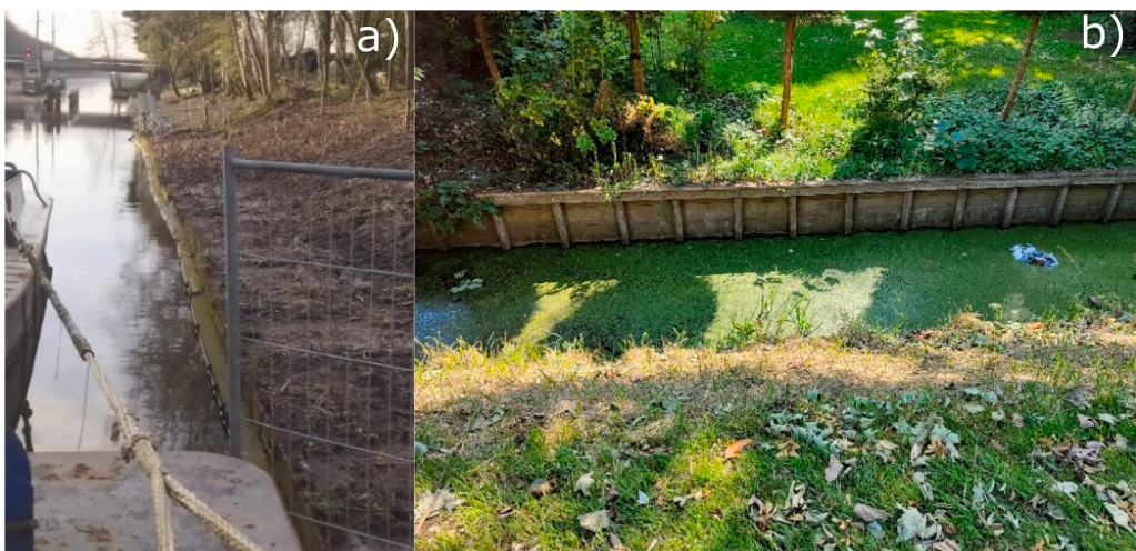
Fig. 1. a) Existing azobé sheet pile nearing end of service life b) Horizontal wooden elements protecting bank of the canal.
