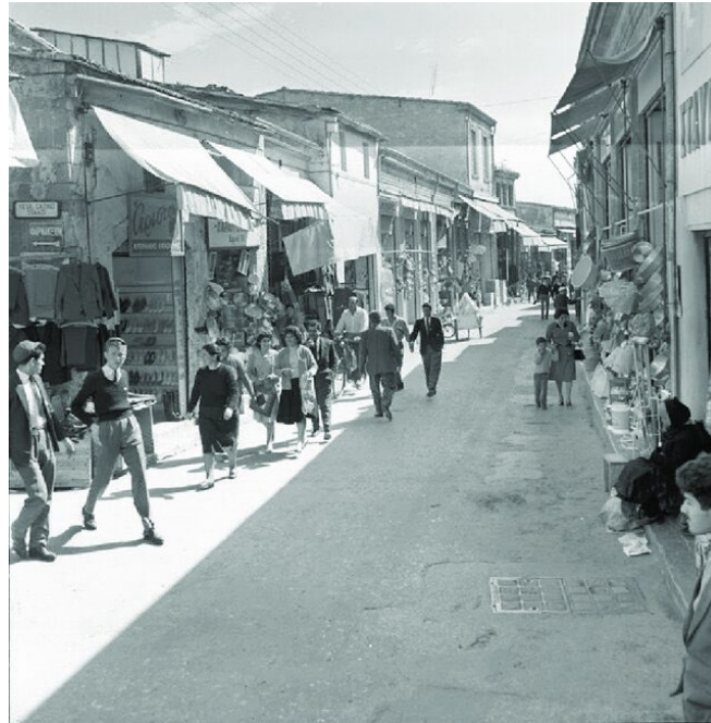
Figure 14: Hermes Street near Platanos Opposite Sophianos—Late 1950s, photograph, Press and Information Office Archive, 20C.151 (20), Ministry of the Interior, Republic of Cyprus, uploaded by Anita Bakshi, in Remains of the Day , https://www.researchgate.net/publica
