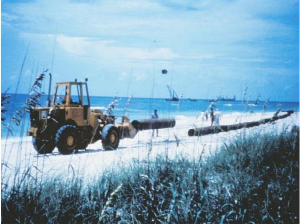
Machinery works on the beach to connect the pipeline segments while offshore dredge and support vessels can be seen in the top right section of the photograph. This is from the 1984 beach renourishment project.
