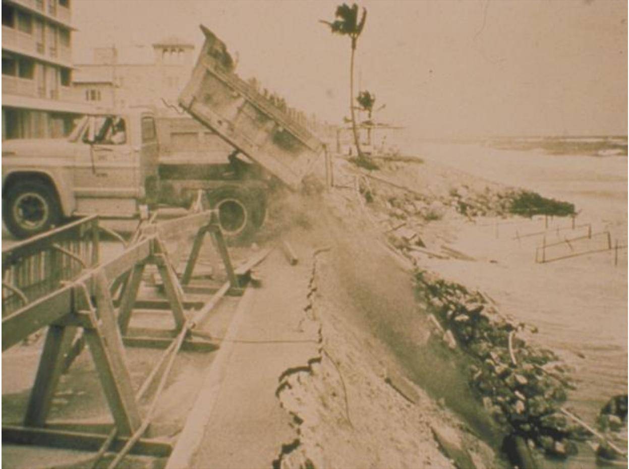
In response to erosion problems and rocks were thrown in the base of the eroded dune with no design criteria, late 1960s to early 1970s.
