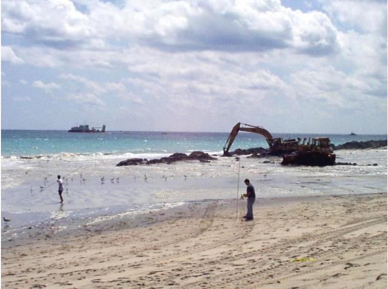
Beach view of the 1992 beach renourishment project, dredge is offshore in the top left, machinery distributes the sand on the beach and surveyors verify the elevation of the fill.
