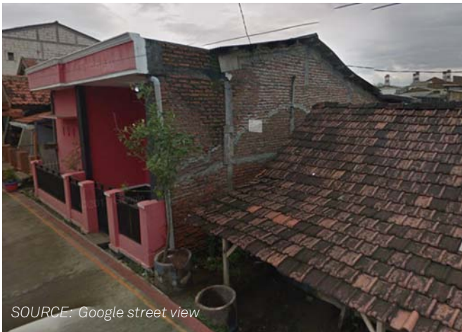
Rebuilding house on old structure
