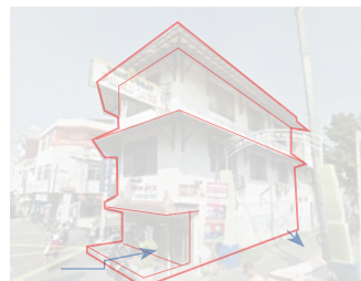
The major house in Pecinan regard water side as a rear side, with close wall or small rear doors.
