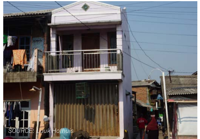
Rebuilding house on old structure
