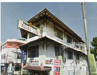
3. Shop+Resident Water next to the water front in Pecinan's boulder.
