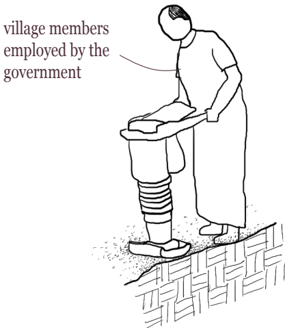
a compacted with hand-held rammer
