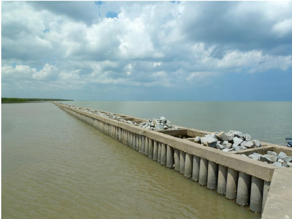
Figure C.2: Concrete breakwater along west coast of Cà Mau (photo taken by author during field trip in May 2016). In the third compartment from bottom right, the rock filling has been removed to allow for sediment transport.
