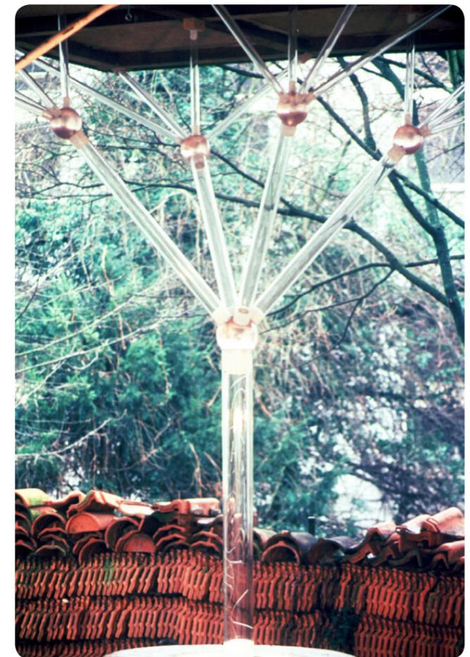
Fig. 03.3 l: Tree shaped structure in Glassbaum, Aachen (Glasbaum 2013)
