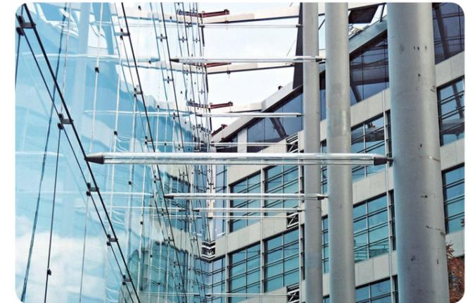
Fig. 03.3 k: Glass tubes used in facade structure of Tower Place, London
