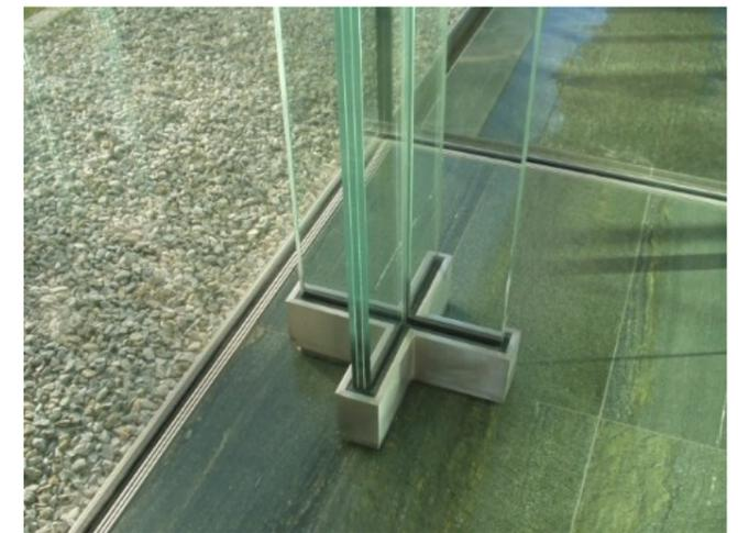
Fig. 03.3 g: Cruciform Profiled column at Danfoss Headquarters in Denmark (anne bagger 2009)
