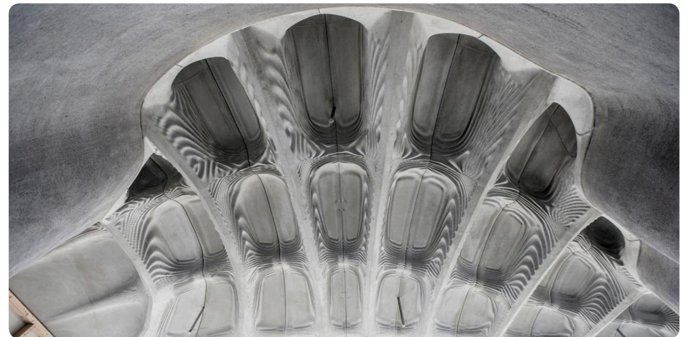
Fig. 03.6 i: 7.4 m long optimized concrete slab casted in 3D printed sand mould. (The Smart Slab n.d.)
