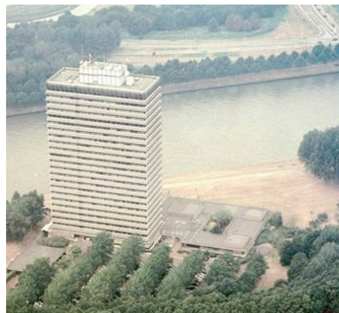
6.03 The westraven before the renovation
