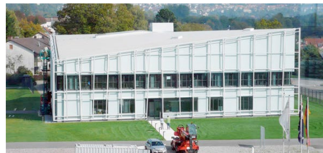
5.03 Inner façade is showing during construction
