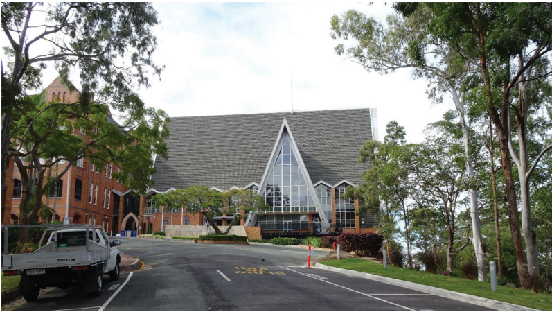
Figure 10. Recent exterior photograph of Stuartholme Catholic Girls School Chapel, Toowong (1963), by Leo Drinan of Hennessey, Hennessey and Co. (Daunt, 2018).
