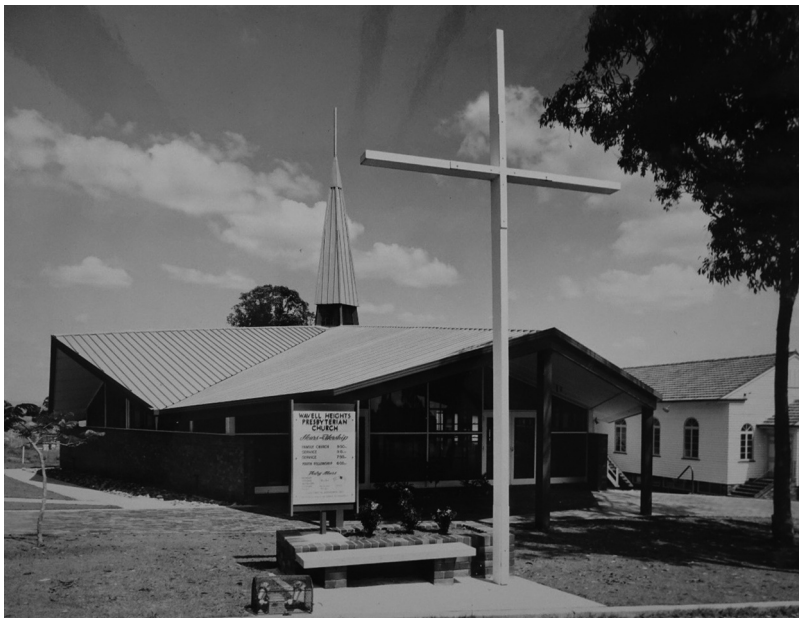
Figure 16. Exterior view of St Luke's Presbyterian Church, Wavell Heights (1966), by Cross and Bain, photographed on the opening day (photographer: L. & D. Keen Pty Ltd. 1966, courtesy Wavell Heights Presbyterian Church).
