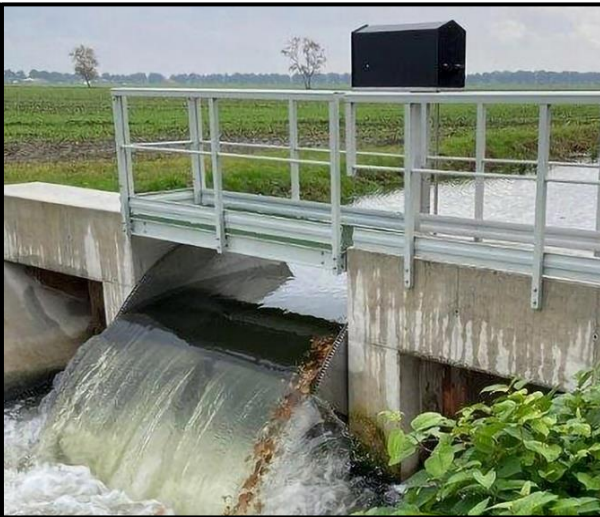
Figure 7 - An adjustable tilt weir (Dutch: “kantelstuw”) in a channel along the Kamperhoeve street in Hattem, NL, located here . Image referenced from local newspaper Nieuwsblad Schaapskooi .
