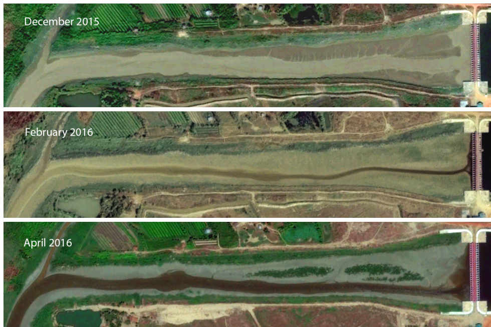
Figure 2.2: Google satellite images of the upper part of the creek near the Nga Moe Yeik Sluice Gates in the dry season.
