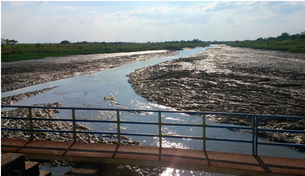
Figure 2.4: Mud deposits in the Nga Moe Yeik Creek as seen from the Nga Moe Yeik Sluice Gates. This picture was taken in May 2016 (with closed gates) and is acquired from Irrigation department after a field visit to the sluice site.
