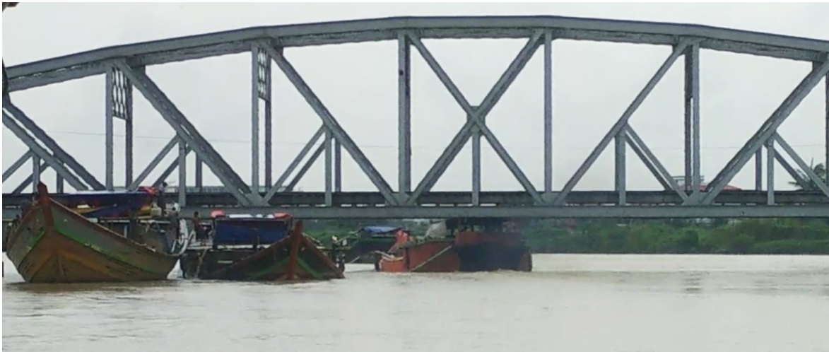
Figure D.2: The last boat of the day just squeezes under the bridge at a location of roughly 17 km from the mouth. Its predecessor wasn't low enough and damaged its wheelhouse after a collision with the bridge. The remaining ships decided to wait for the next tidal window.
