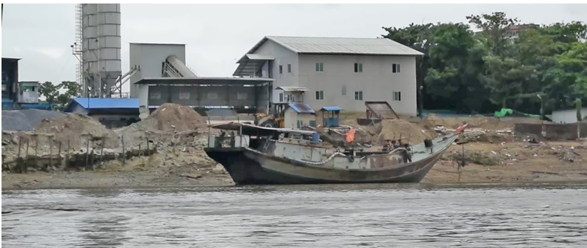
Figure D.3: This dumping site was observed about 1.5 km from the river mouth. During an OBS survey covering 13 hours, several barges have been observed while emptying their holds at this location. To empty the boats hold, use is made of a pump and hose combination to place the sediment behind the wooden structure
