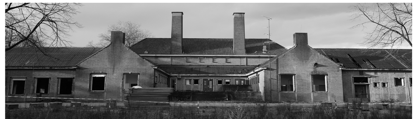
Figure 4: Kitchen building Kolonel Palmkazerne (project site)
