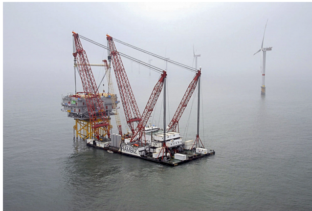
Figure 1.2: Aerial photo of the RAMBIZ 3000 during a substation lift operation
