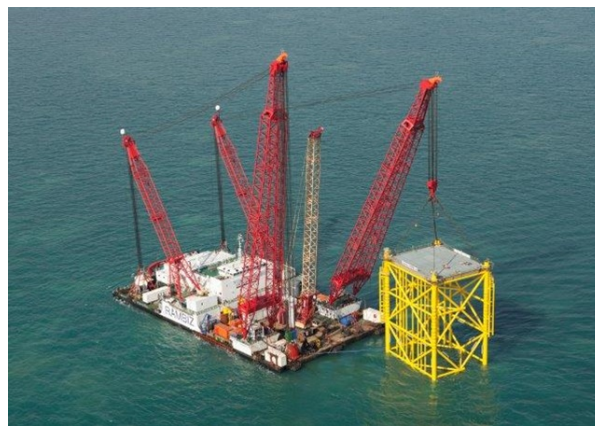
Figure 3.1: Rambiz 3000 during the installation of the Rampion jacket
