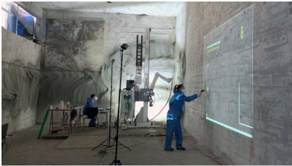
Figure 1: IRoP, interactive robotic plastering system (Mitterberger et al., 2022a).
