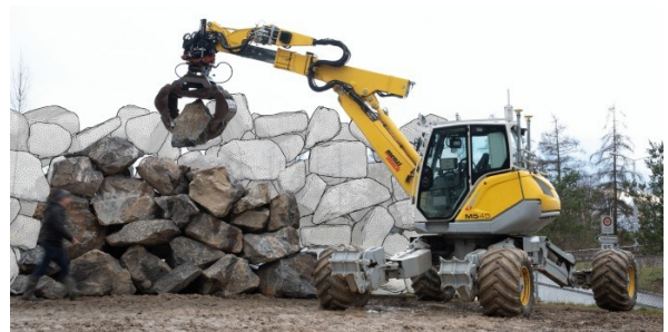
Figure 3: Autonomous Dry Stone Wall Construction (Johns et al., 2020)
