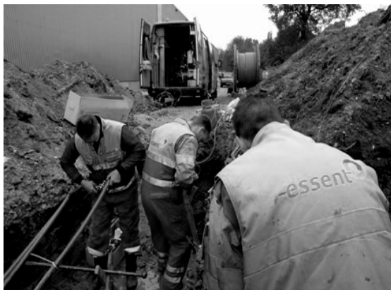
Figure 4.5: Mechanics working in a trench (Werk & Vakmanschap)
