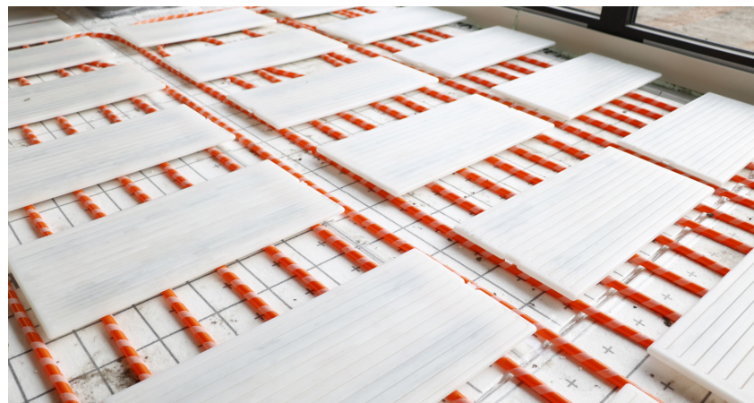
Photo: Floor-heating with PCM elements
