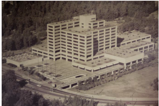
Figure 21: The parking garage is tucked underground with a more subtle car ramp in comparison to City Center & the Toronto City Hall. Helasvuo, Olli, Riikka Koivula, and Tapani Mustonen. “Pohjolan Toimitalo Lapinmäen tie 1.” Arkkitehdit Mustonen , 2013, 30.
