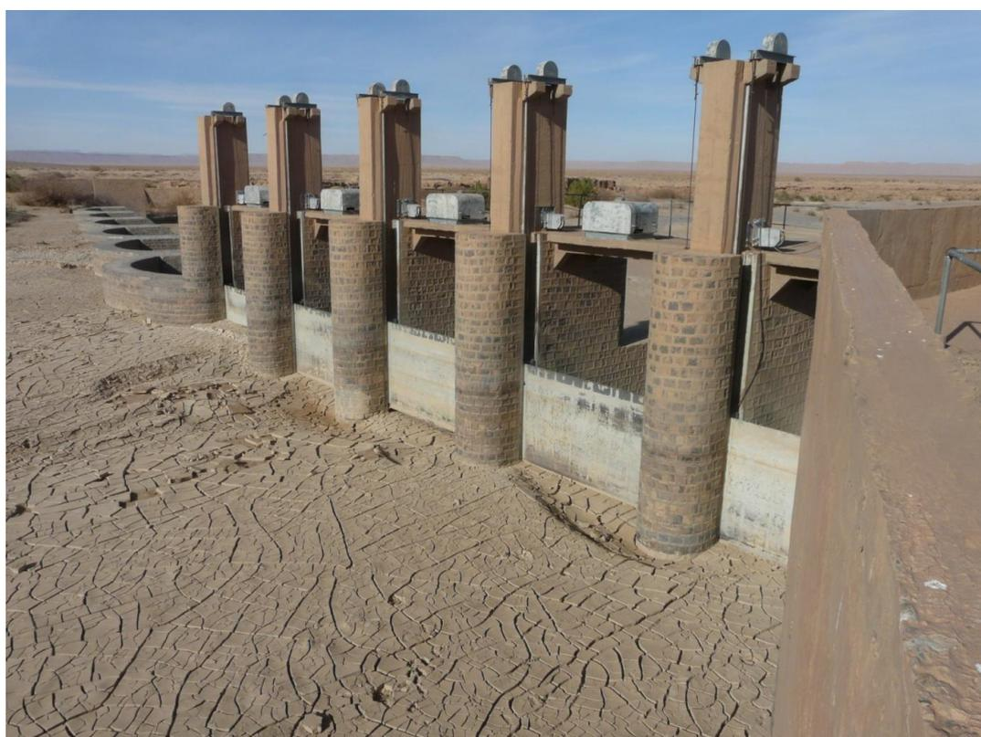
Figure 120: Dam in the oued Rheris, which is also intended to guide the water to the irrigation canals (see location 2a in figure 119).
