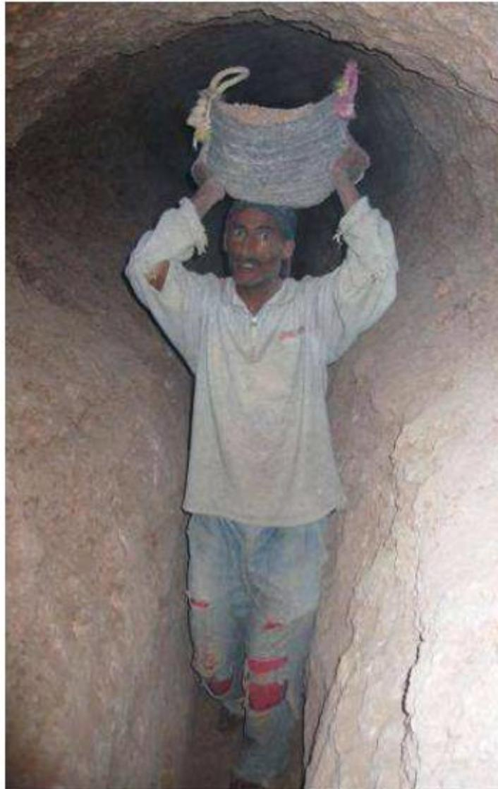
**Figure 33:** Maintenance work in the gallery of a typical khattara (Spoerry, 2007). The canal has on average a width of 30 to 40 cm.
