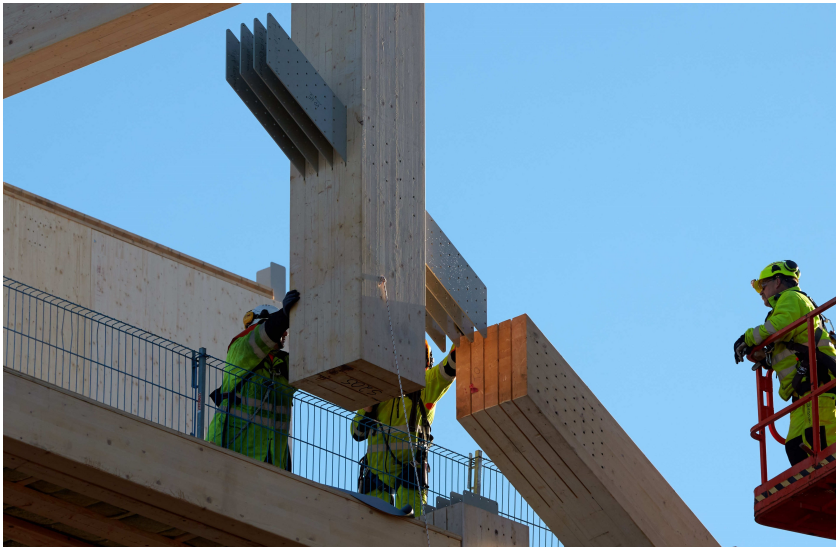
Figure 4.3: Assembly of a truss connection [38, id: 42180].
